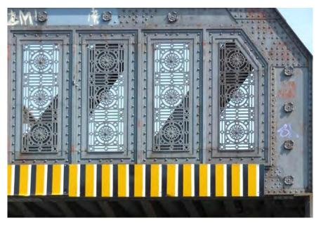
Figure 484 Detail of cast-iron panels
