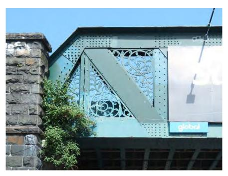
Figure 499 Cast-iron decorative panels at western end of bridge
