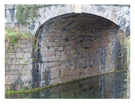
Figure 131 Abutment on southern side of bridge
