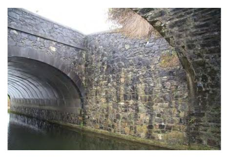
Figure 393 Southern wing wall on eastern side of Mullen Bridge
