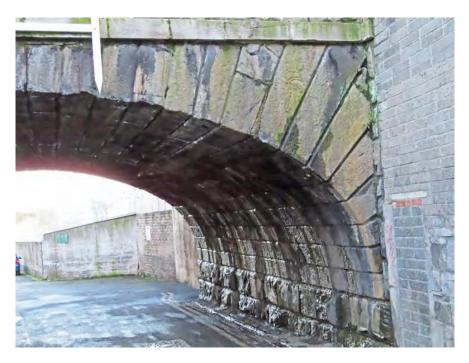
Figure 8 Detail of spandrel and barrel of arch
