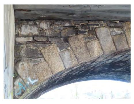
Figure 70 Detail of voussoirs and spandrel on eastern side of Clonliffe Bridge
