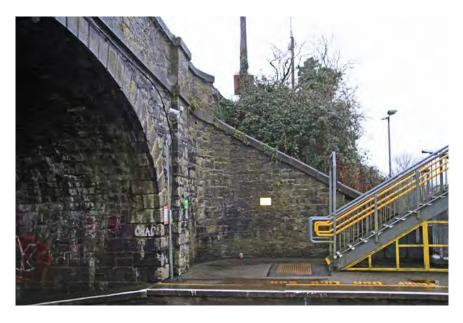
Figure 322 Western wing wall on southern side of railway bridge
