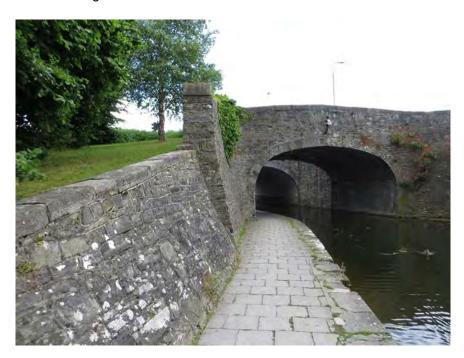
Figure 392 Northern wing wall on western side of Mullen Bridge
