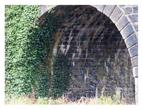
Figure 419 Barrel of vault of railway bridge
