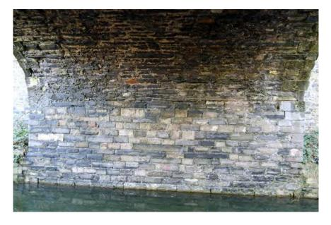
Figure 267 Abutment and barrel of arch
