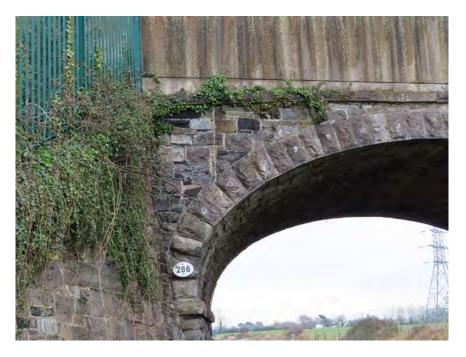
Figure 445 Spandrel at northern end of western arch
