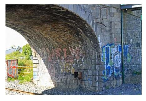
Figure 121 Vault of railway bridge
