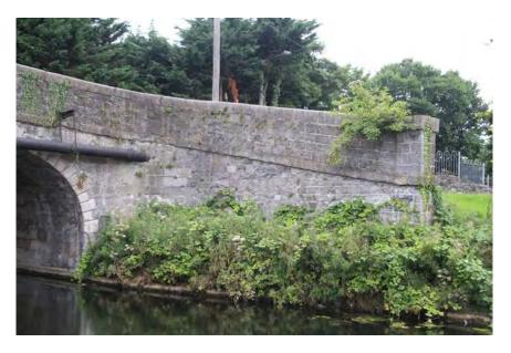
Figure 189 Wing wall on northern side of canal to the east of the bridge
