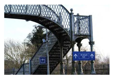
Figure 234 Top flight of stairway and top of trestle
