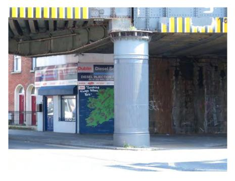
Figure 485 Cast-iron column between the two spans
