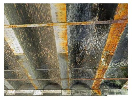
Figure 467 Jack arches on soffit of bridge deck
