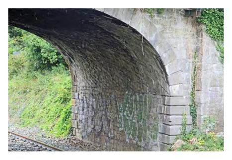
Figure 198 Abutment and soffit of bridge on southern side
