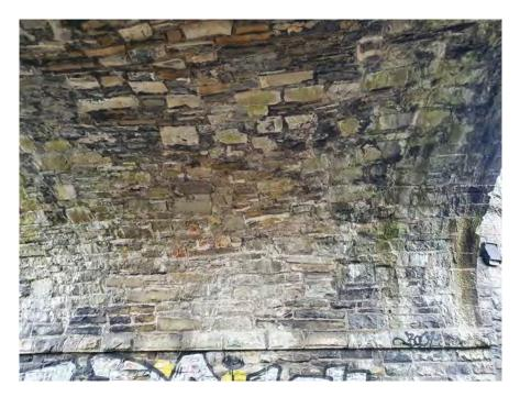
Figure 450 Barrell of vault of Barnhill Bridge
