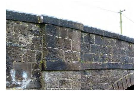
Figure 426 Pier between railway and canal on western side, with string course and coping stones
