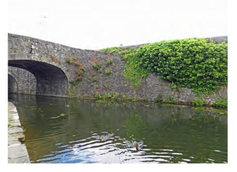
Figure 391 Southern wing wall on western side of Mullen Bridge
