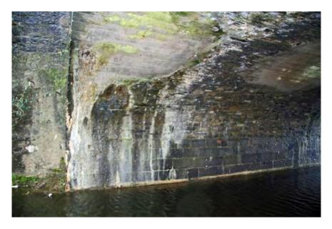
Figure 335 Abutment and spring of vault on eastern side of bridge
