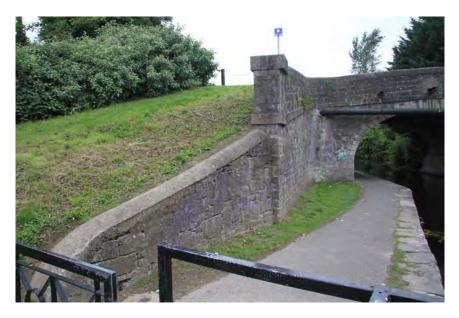
Figure 190 Wing wall and retaining wall on southern side of canal to the east of the bridge
