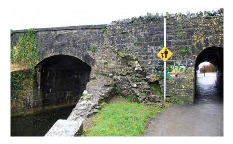
Figure 414 Remnant of original wing wall
