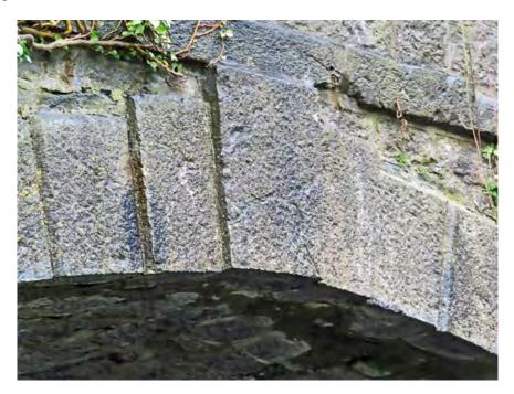
Figure 224 Detail of keystone on eastern side of bridge
