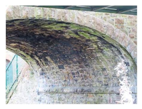
Figure 456 The arch ring and the barrel of the vault of Dunboyne Bridge
