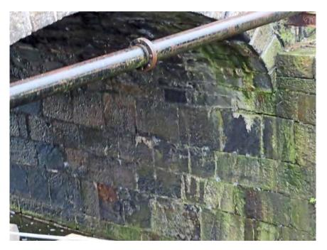
Figure 147 Abutment and spring of arch on southern side
