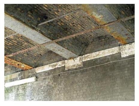
Figure 473 Padstones and string course beneath beams
