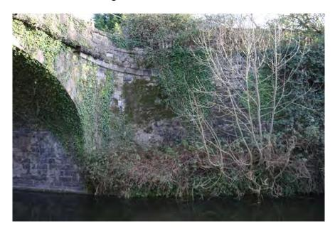
Figure 279 Wing wall at south-western side of bridge
