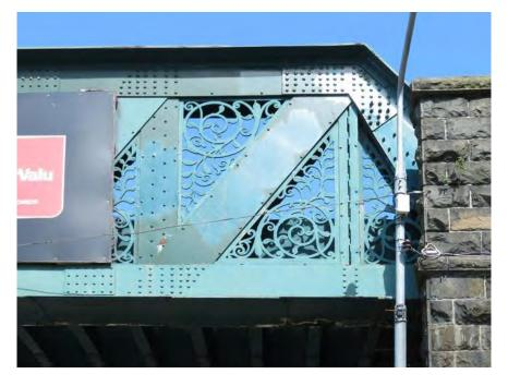
Figure 498 Cast-iron decorative panels at eastern end of bridge
