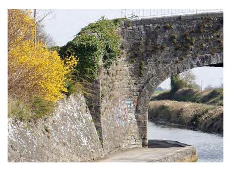
Figure 367 Western wing wall of canal bridge
