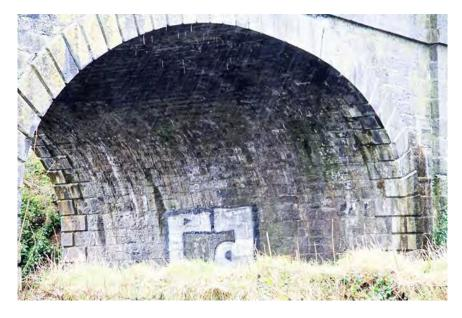
Figure 373 Barrel of vault of railway bridge
