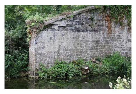
Figure 291 Southern wing wall on eastern side of bridge
