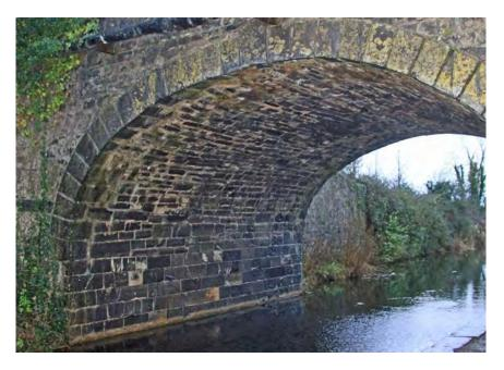
Figure 293 View into bridge showing masonry of barrel
