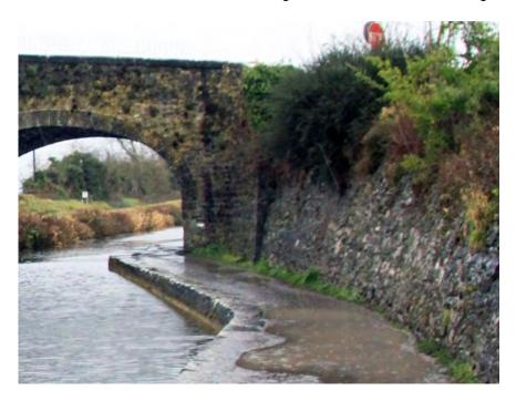
Figure 368 Eastern wing wall and retaining wall of Canal bridge
