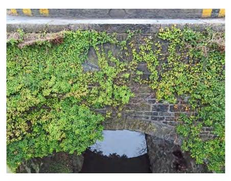
Figure 210 Eastern keystone and parapet
