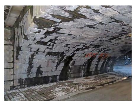
Figure 14 Barrel of masonry arch at southern end of bridge
