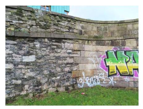
Figure 50 Junction between wing wall and retaining wall on eastern side of bridge
