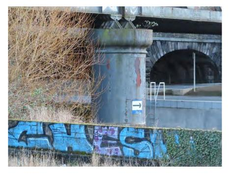
Figure 23 Detail of cast-iron pier
