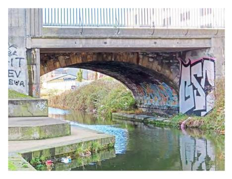
Figure 68 Eastern elevation of Clonliffe Bridge, showing masonry arch
