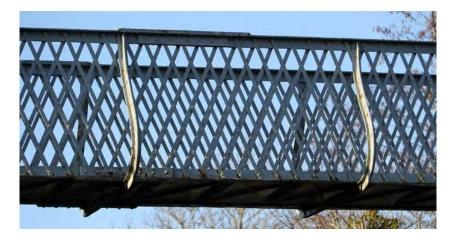
Figure 238 Outer face of parapet on bridge deck
